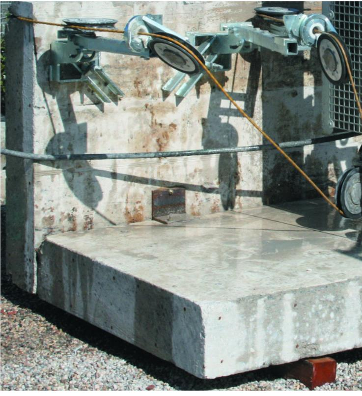
structures. The conventional tools require slow paces and in most cases is necessary a large manpower force and a very expensive environmental clean-up. Deconstruct the concrete in an ecological way means acting without interrupting productive activities, with total absence of vibrations and low noise level.
