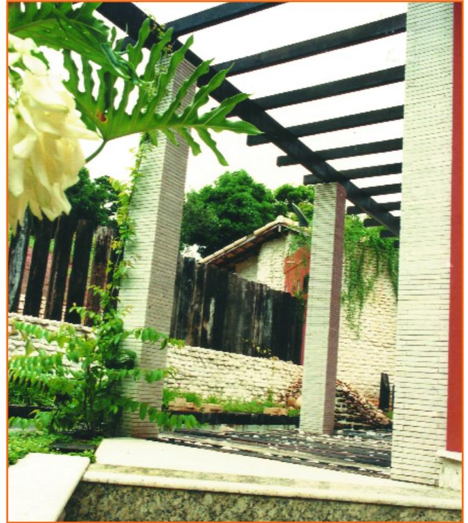
Column: using the leftover of granite with the irregular face to in. Cutting first at the right size. Like revestment or like shape
