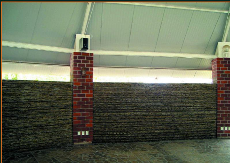
Panel: left over with mortar, one on top of the other, irregular face out. If burned with fire, they become homogeneous
