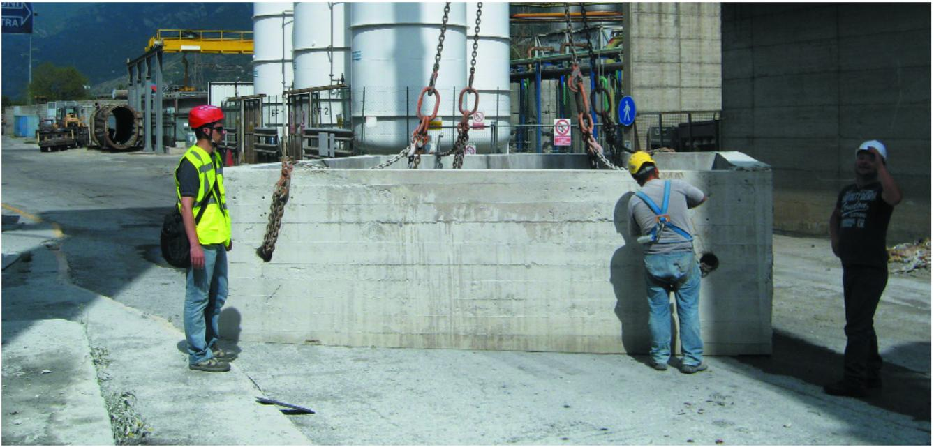
due to falling materials. As it was too expensive to cover the pipes with a temporary protective structure, it was agreed with the customer to perform the demolition work in a short span of time during which, for other maintenance work, the plant was stopped, the pipes drained and then carefully secured.
